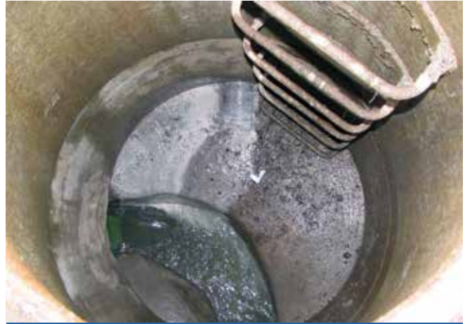
Photo showing the prebenching of the manhole with sewage channel.
