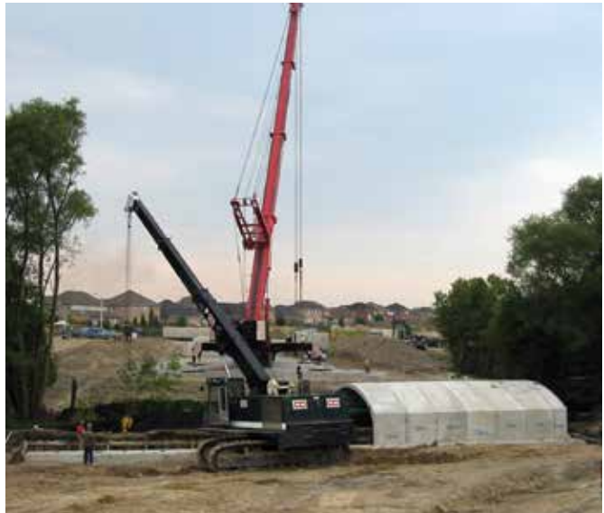
Installation of precast footings and CON/SPAN units for large culvert over Stouffville Creek.
