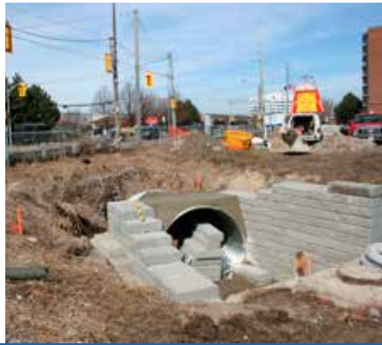
Corrugated steel arch culvert extension encased in concrete to accommodate vehicular access to Birchmount Road.
