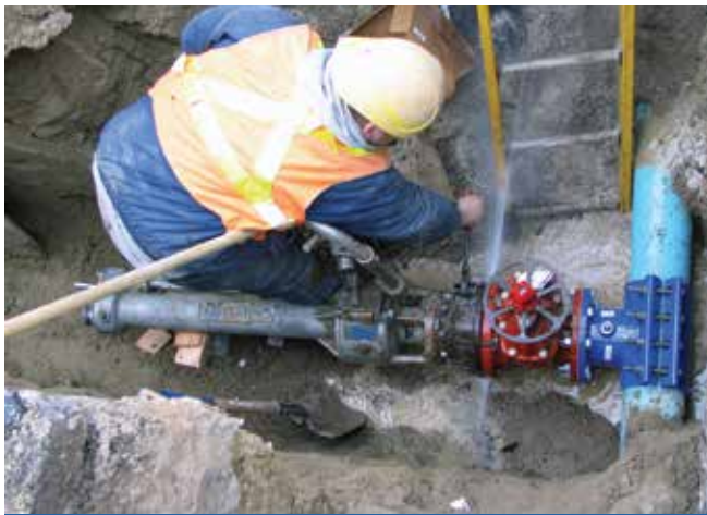
New hydrant installation on a new watermain.
