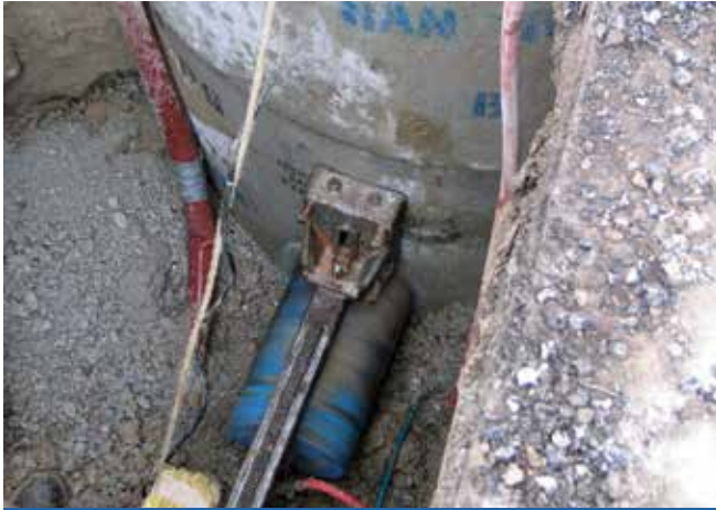
Coring concrete into existing manhole for new sanitary sewer connection.
