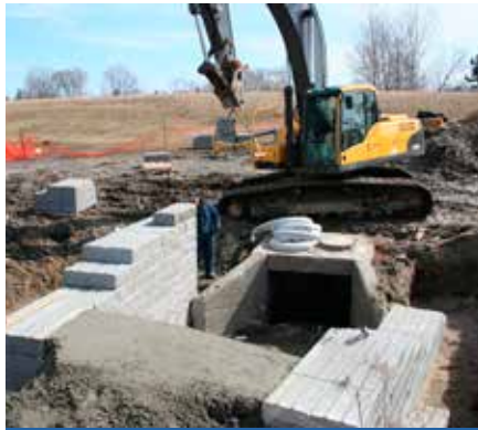
Corrugated steel arch culvert extension encased in concrete to accommodate vehicular access to Birchmount Road.
