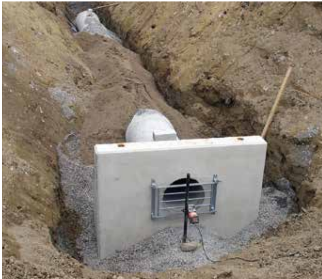
Construction of precast concrete pipe storm sewer.
