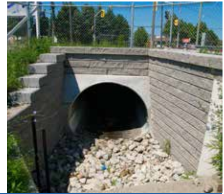
Corrugated steel arch culvert extension encased in concrete to accommodate vehicular access to Birchmount Road.
