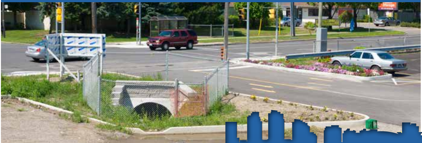
Corrugated steel plate culvert under Birchmount Road after the extension of Comstock Road.
