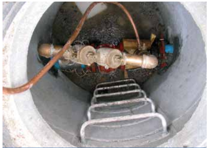
New backflow prevention device in structure.
